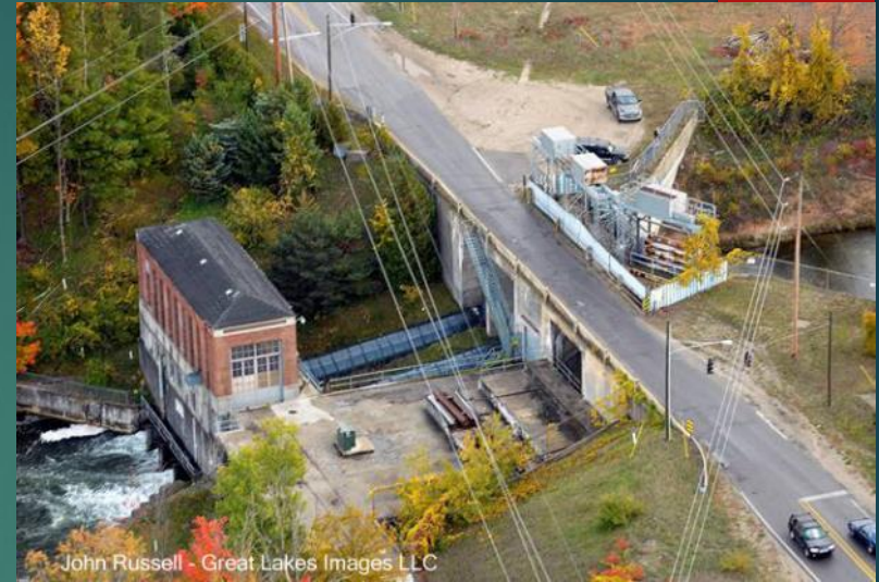
#2 Boardman & Cass Road Bridge
