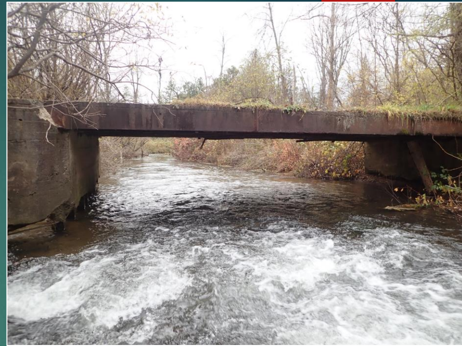
Downstream of the triple culverts.
