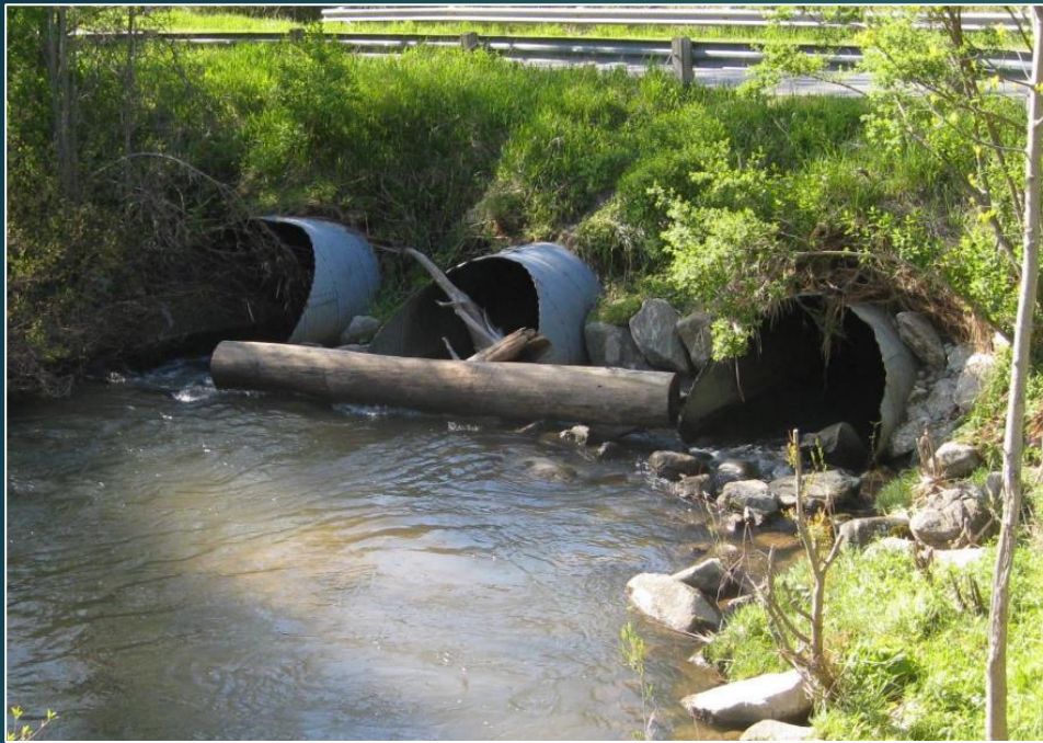
Downstream of the dam.
