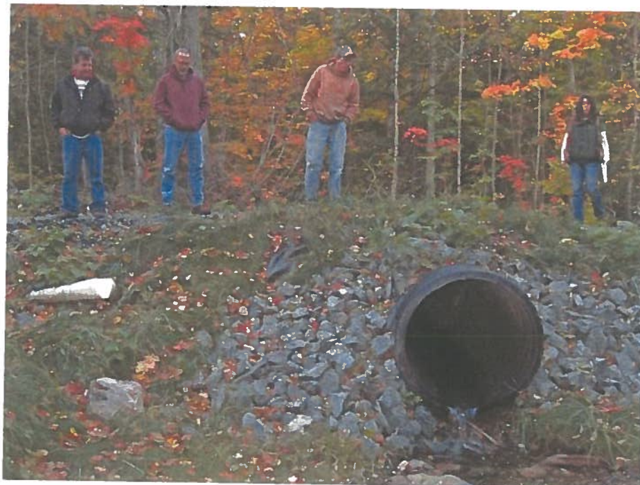
Auditors discuss perched culvert placed over bedrock.
